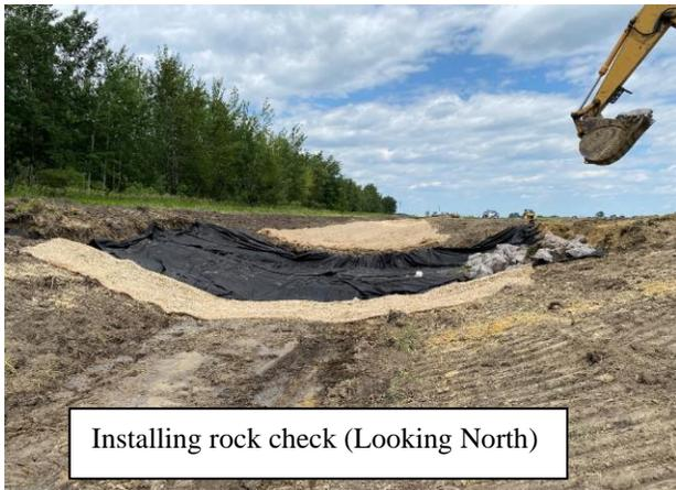
Installing rock check (Looking North)
