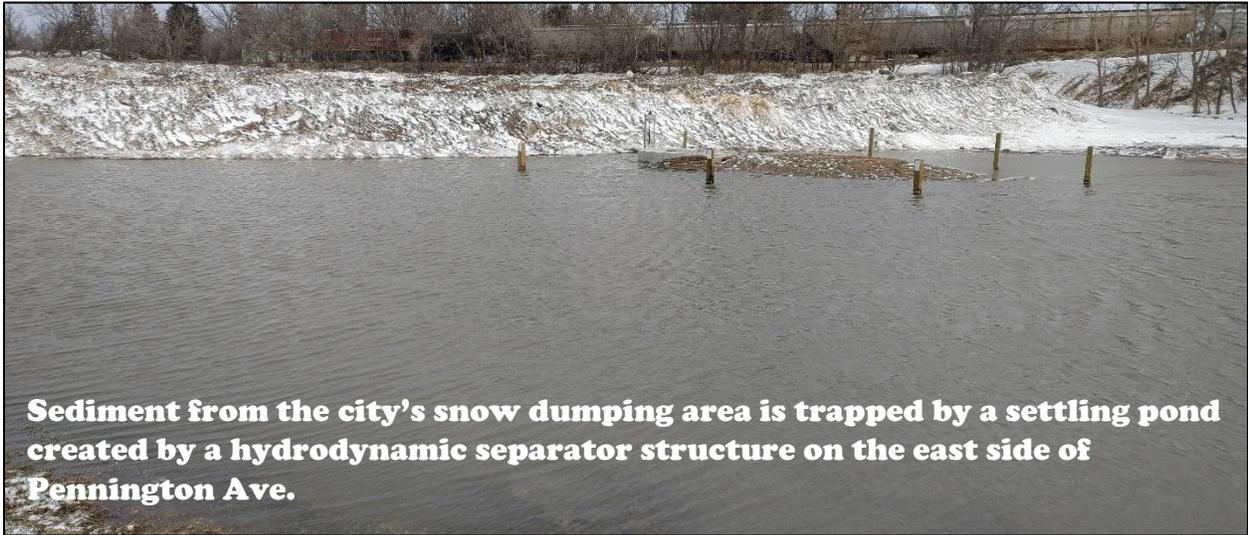
**Sediment from the city's snow dumping area is trapped by a settling pond created by a hydrodynamic separator structure on the east side of Pennington Ave.**
