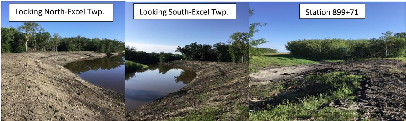
In the recent years, sloughing along the system has increasingly gotten worse. There were 2 locations that had sloughing fixed on the system that was paid by one watershed one plan (1W1P). Both locations had toe wood sod mat installed to help prevent undercutting and sloughing. There are pictures of this installation on the next page below the chart. See also 1W1P projects for more information.
