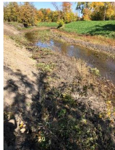
These photos are areas along State Ditch #83 that were part of the Toe Wood Sod Mat Installation. It was installed to protect the integrity of the ditch bank and stop or slow down bank sloughing and erosion.
