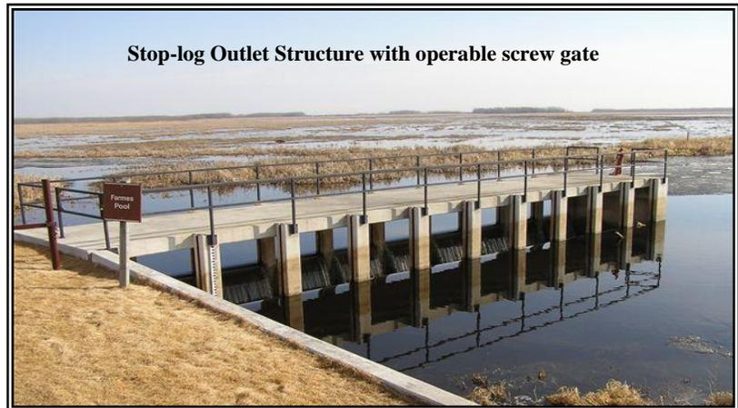
**PROJECT COMPONENTS:** Approximately 9 miles of earthen embankment, an outlet control structure, rock lined emergency spillway, and an enlargement of a portion of Ditch 200.
