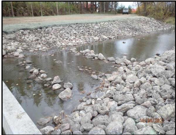
Riprap riffles downstream of concrete structure
